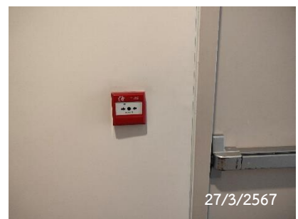
Fire Alarm Manual Station
